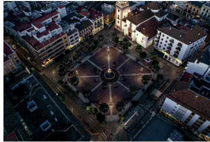
Figure 8: Lighting renewal project in Algeciras, Signify.
